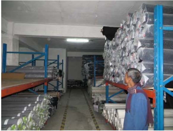
P 12.3 Inadequate clearance from ceiling
