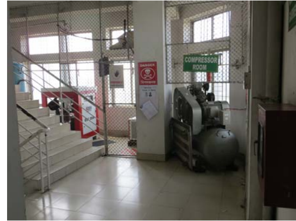
P 11.3 Obstacle in Stairway
