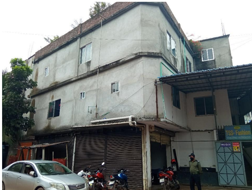
Figure 5: Exterior View of Factory Building
