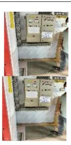
পরিদর্শন | Cable ends not properly or crimped || Connection without lug || Undressed messy wire inside || Door not earthed || No clear identification mark on distribution board || Loose Circuit Breaker
