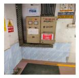
No instruction for first aid to electrical shock and artificial respiration \( \) Non-conductor পৰিদৰ্শন without lug \( \) Access obstructed to substation equipment \( \) No fire rated enclosure from floor to ceiling
