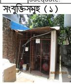
পৰিদৰ্শন Location – Generator room – Proper working clearance was not maintained around the প্ৰব্বেষ্ণন generator.
