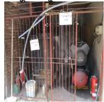
পরিদর্শন Location – Generator room – Fire protection were not provided (Heat detector and পর্যবেষ্ণণ smoke detector) in Generator rooms.
