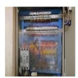
পরিদর্শন "Distribution board, 4th Floor (including panel door) and metallic cable channels in পর্যবেষ্ণন the building are not connected to the earthing system. "
