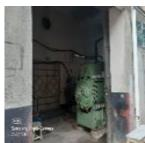
The generator room is not properly segregated from the rest of the occupancy due to প্ৰিদৰ্শন presence of non Fire-rated Door □No detector in generator room □Combustible/junk materials inside generator room □ One point frame earthingof generator instead of two No detector in generator room
