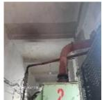
া The generator room is not properly segregated from the rest of the occupancy due to পৰিদৰ্শন presence of non Fire-rated Door □No detector in generator room □Combustible/junk পৰ্যবেষ্ণনা materials inside generator room □ One point frame earthingof generator instead of two No detector in generator room
