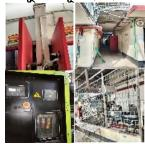
The generator room is not properly segregated from the rest of the occupancy due to presence of non Fire-rated Door .
