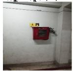
পরিদর্শন Location– 1st floor The water throw of jet is around 20 ft distance. Hose pipe water পর্যবেষ্ণন pressure is lower than the minimum requirement of RMG guideline.
