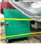
পৰিদৰ্শন Location – All distribution board – Earth Continuity Conductor (ECC) was not adequate প্ৰ্বৰেষ্ক্ৰণ & dedicated to circuit.
