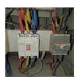
Location - Changeover at Generator room, Shed - 1, LT panel at LT room, Shed - 1, DB প্রিদর্শন at Shed - 2, DB - 2 at Ground floor, Main building, DB - 2 at 1st floor, Main building, DB - 3 at 1st floor, Main building - Looping, Bunching at MCCB/MCB and Bus bar terminal were observed.
