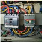
পরিদর্শন Location – All distribution board – Wiring diagram / circuit list were not available on all পর্যবেষ্ণন Distribution Board. In some DB's circuit list was available but mismatched.
