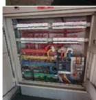
পরিদর্শন Location - Office room - Periodical inspection and testing (insulation, earth resistance, পর্যবেষ্কণ operation test) of all electrical equipments was not done.
