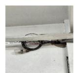
পরিদর্শন Location – LT panel at LT room, Shed – 1 – Cables / wires and MCCB weren't selected প্র্যবেষ্ণ্যণ with suitable rating for desired application.
