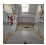
Location-Stair-2 south side at building 1 Stairways are finished near to final exit gate at ground floor. But after that, it meets the final evacuation passageway which is not fire separated corridors adjacent to the ground floor production areas windows and store room exit.
