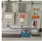
পরিদর্শন Stranded conductors are not provided with proper cable terminator (cable sockets, প্র্যবেষ্কণ sleeve or ferrules, etc.). Location: MDB/ Finishing Section/ Ground floor.
