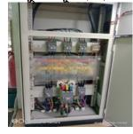
পরিদর্শন Distribution boards are not marked separately for lighting and power circuit. Location: পর্যবেষ্ণণ DB-1/ Sewing Section/ Ground floor, DB-2/ Sewing Section/ Ground floor.
