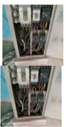
পরিদর্শন পর্যবেষ্ক No instruction for first aid to electrical shock Access obstructed/barred Connection without lug Undressed messy wire inside Body & door not earthed Installed on wooden board MCCB/MCB box broken/loose Does not have duplicate earth leads
