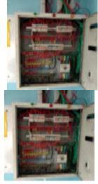
ll No instruction for first aid to electrical shock ll Access obstructed/barred ll প্রিদর্শন Connection without lug ll Undressed messy wire inside ll Body & door not earthed ll প্রবিশ্বন Installed on wooden board ll MCCB/MCB box broken/loose ll Does not have duplicate earth leads
