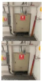
Does not have duplicate earth leads 01–09–2022 visit observation: 1.Panel board were not install properly. 2.Duplicate earth leads were not provided in MDB. 3.Body & door earthing were found in distribution boards. 4.No visible burn were observed. 5.Clear identification mark on distribution board were not found. 6.MDB/SDB/SB or MCB were installed on metal
