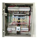
পরিদর্শন Multiple connections of cables at busbar terminal and circuit breaker terminal are পর্যবেষ্কণ observed within distribution boards.
