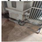
পরিদর্শন Each applicable circuit is not provided with dedicated neutral. There is no marking to প্রবিষ্কণ identify neutral cable for specified circuit.
