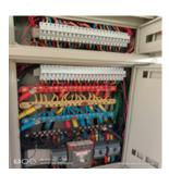
পরিদর্শন Location–All panels –Earth Continuity Conductor (ECC) was not provided adequately পর্যবেষ্কণ & dedicated to circuit.
