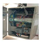
পৰিদৰ্শন Location–Most of the Distribution Board –Bunch of cable was observed inside the প্ৰ্ববেষ্কণ panels at most of the distribution board.
