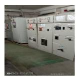
পৰিদৰ্শন Location–Substation room at Ground Floor, Utility Building – All incoming and outgoing প্ৰ্ববেষ্কণ circuits of HT and LT panels was not clearly and permanently labeled for identifications. ক্যাপ আইটেম ক্যাটাগৰি
