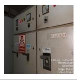
পৰিদৰ্শন Location–Most of the Distribution Board ––Cables / wires and MCB/MCCB was not প্ৰবিষ্কৃত্য selected with suitable rating for desired application at most of the distribution board.
