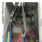
পরিদর্শন Location–Most of the Distribution Board –Earthing connection was not provided at the পর্যবেষ্ণন panel door at most of the distribution board.
