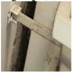
Temperature differences of 21°C to 40°C were observed based on comparisons between component and ambient air temperatures Probable causes are loose connection, over loading, multi cable at single point, rusted connection, use of improper lug, improper cable joint, improper cable bending, damage insulation, internal problem etc.
