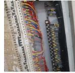
পরিদর্শন List and diagram of the circuits are not available for distribution boards. Also there are পর্যবেষ্ণন no means of identification mark for cables.
