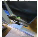
পরিদর্শন Each circuit is not provided with dedicated earthing and there is no marking to identify পর্যবেষ্ণন earthing cable for specified circuit.
