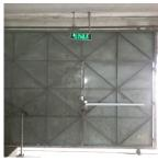
পৰিদৰ্শন Location – All exit doors in egress route The egress route exit doors are sliding type and প্ৰবিষ্কা there is chance that doors get locked due to any obstruction in opening/closing.
