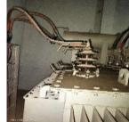
া The generator room smaller than the required size i Inadequate ventilation of the generator room is not properly segregated from the rest of the প্ৰব্ৰেষ্ণ্ৰ occupancy due to presence of non Fire-rated Door i No appropriate detector in generator room One point frame earthing of generator instead of two
