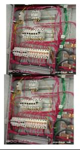
পরিদর্শন Without lug 🛘 Undressed messy wiring/cables 🖟 Cable ends not properly soldered or crimped
