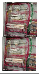
পরিদর্শন Without lug 🛘 Undressed messy wiring/cables 🖟 Cable ends not properly soldered or crimped
