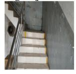
পরিদর্শন Location – Stair – 2 and stair – 3 Collapsible doors are installed, which are without self প্রবিষ্কণ closing type at evacuation route, so stairs require fire rated self – closing door.
