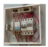
Location-MDB in Generator room, DB in Fabrics Section, DB in Cutting Section, DB in Sewing Section (South), DB in Sewing Section (North) - Wiring diagram/ circuit list was not available on every Distribution Board.
