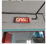
পরিদর্শন Location: All occupied floors At every floor, sufficient number of emergency lighting are প্রবস্থেপ not provided for evacuation pathway.
