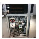
panel. 4. Well dressed cabling with lugs is not ensured.
